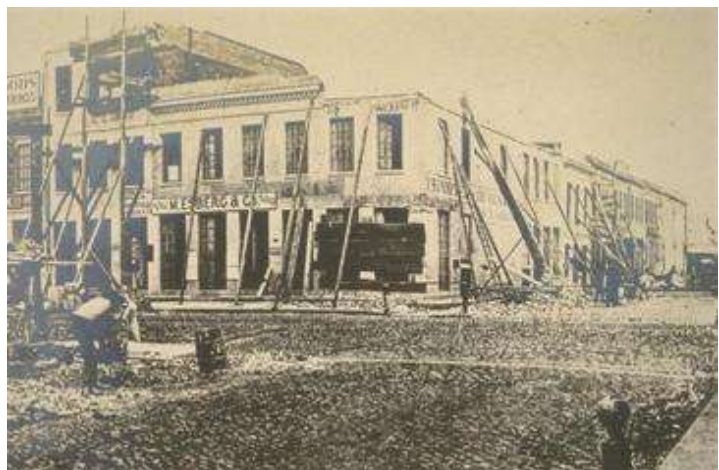
Battery St. (courtesy Bancroft Library)
