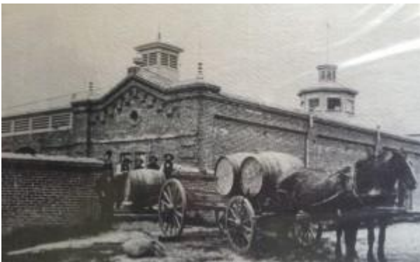
Figure 4 East-side of the Gallegos- Palmdale winery.
