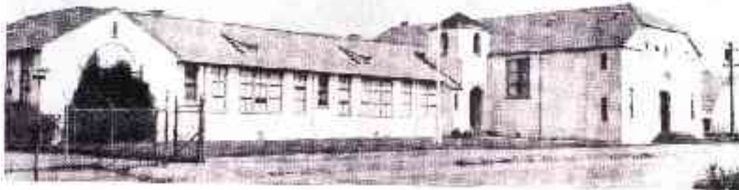
(Decoto Elementary School and Auditorium)
