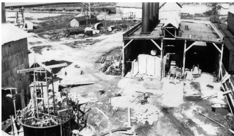
Demolition of old boiler room (note the smoke stacks)
