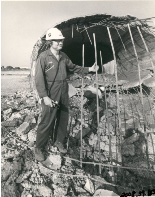
View of demolished smoke stack from its base
