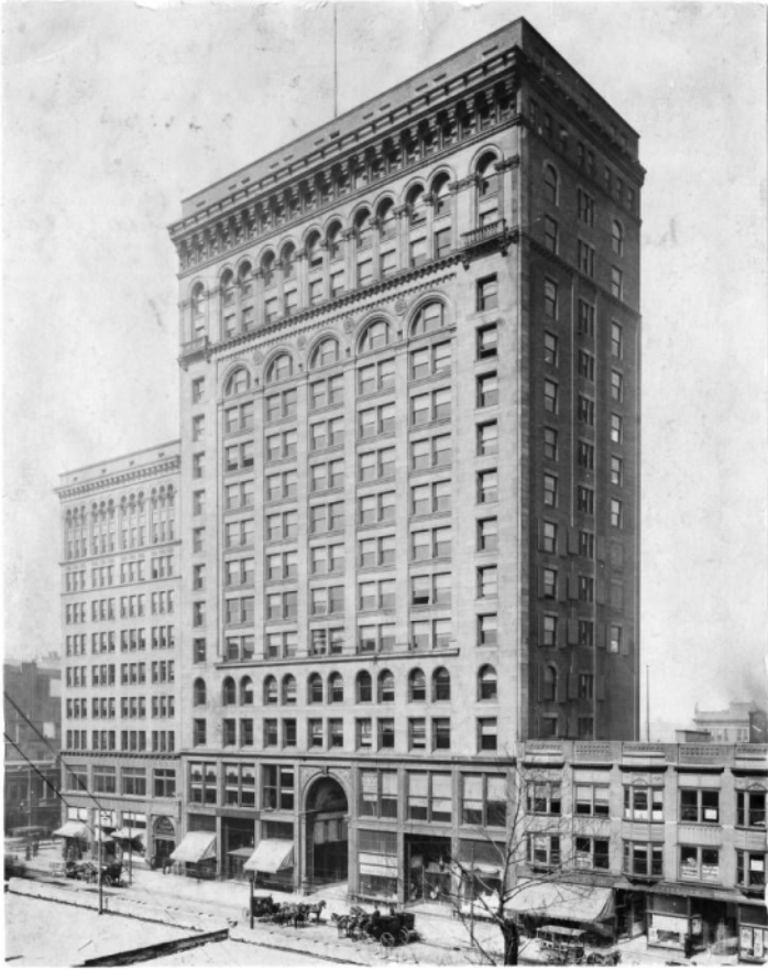
New England building on Euclid Ave, in Cleveland, Ohio. E. H. Dyer & Co. had offices in this building in 1903. (Courtesy of the Cleveland Public Library)
