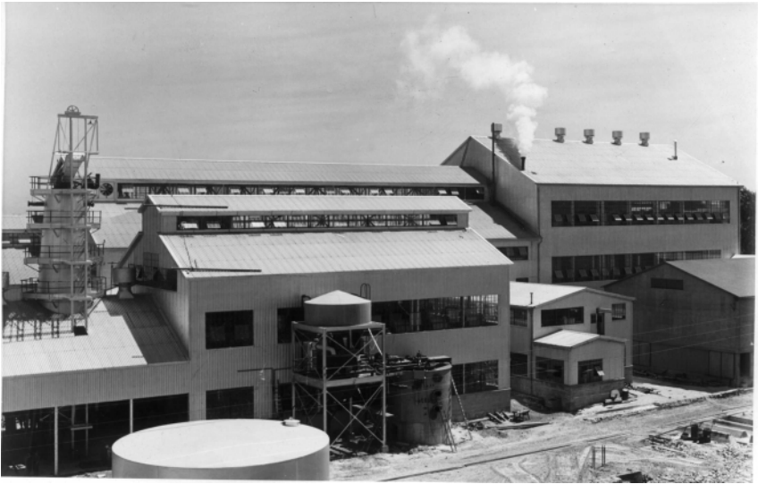
New metal factory almost finished
