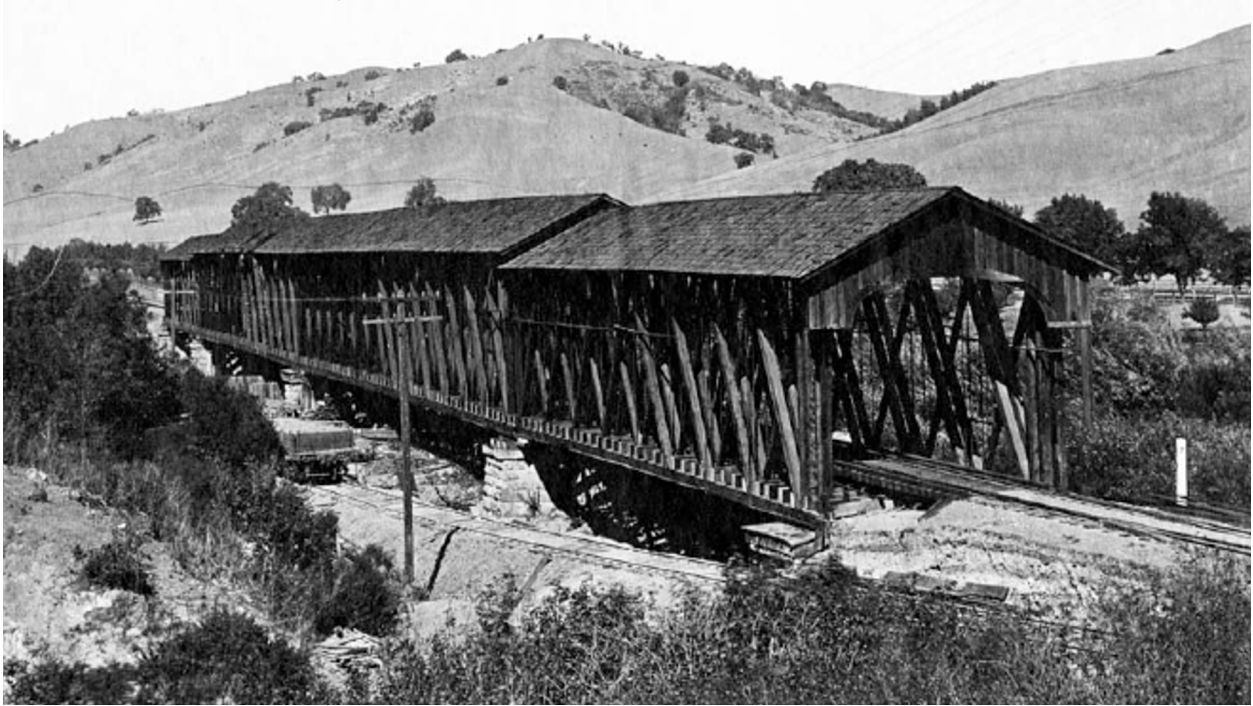
Fig. 8. The Arroyo de la Laguna Bridge (MP 36.87, looking northeast) -- the fourth bridge up Alameda Cañon along the WPRR line. Although it was more than four miles up from where the Cox tracklayers stopped at the San José 20-mile mark (MP 32.75), it appeared that the Cox masons continued their work further upstream and completed the stone piers and abutments of the fourth bridge. Thus, the original Arroyo de la Laguna Bridge was a structure built by two different gangs: the Cox gang built the stone piers and abutments in 1866 and in 1869 the Ryan gang built the rest of the superstructure on top of the stone infrastructure.
