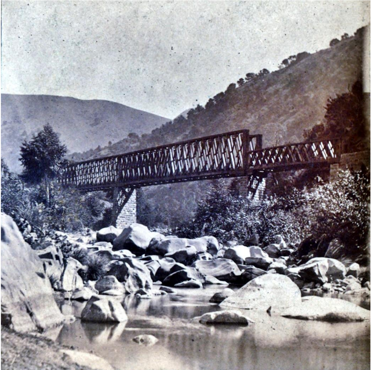
Fig. 5. The Cox gang built “three very large massive bridges, built of the very best [wooden] material, on solid stone masonry.” This photo is of the third bridge, Farwell Bridge, which is still in use (as well as the second bridge, Dresser Bridge). Over the years, the Farwell bridge’s superstructure was replaced with steel ones, but it was, and still is, supported by the original 1866 solid stone piers.
