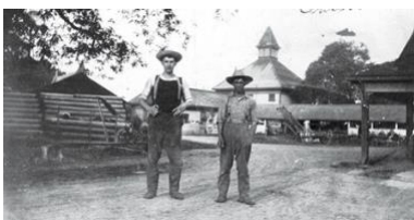
Workers at Innes-Cloverdale Ranch in Centerville with the carriage house in the background. (AB1)
