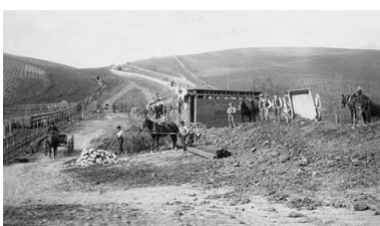
Road crew cutting down a hill near a cemetery on road from Mission San Jose to Warm Springs (AB4)
