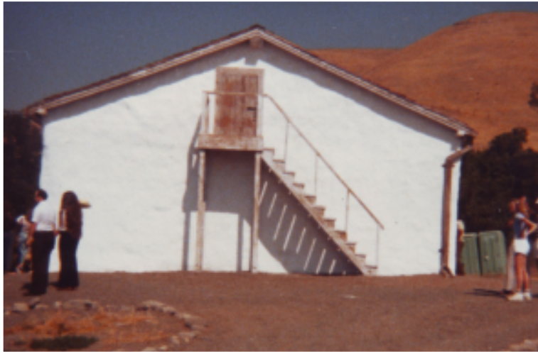
Exterior of west end of Adobe, showing stairway to the second floor.
