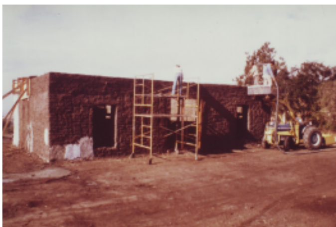
The Adobe during the process of restoration.
