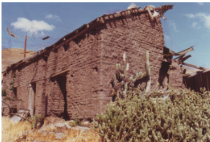
Close up of condition of Adobe before restoration.
