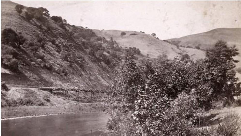
Fig. 6. Card 1516: Alameda Creek and Cañon, Central Pacific Railroad. Shows the intact Vallejo's Mill trestle flume on the bank across the creek, which is the alignment of the new mainline to be constructed by Central Pacific. Note the man standing on the near shore; likely the photographer's assistant to call attention to the flume across the creek. Image courtesy of the Society of California Pioneers, SCP-1245; cropped by the author to show the man.
