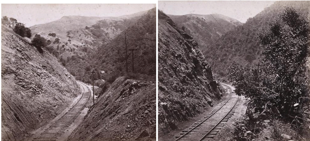
Fig. 12. (a) Left. Card 1529: The Big Cut, above Third bridge, Alameda Cañon. (b) Right. Card 1530: The Big Cut, above Third bridge, Alameda Cañon. Shows the treacherous landslide-prone slope on the outside of the curve (left), and the steep rock-cut on the inside of the curve (right), both hand-carved precisely by Chinese builders to maintain mainline grade and curvature on a horseshoe curve, pictured before the outside slopes were removed likely by machinery in the early 20th century. Images courtesy of the Society of California Pioneers, SCP-1258, SCP-1259.
