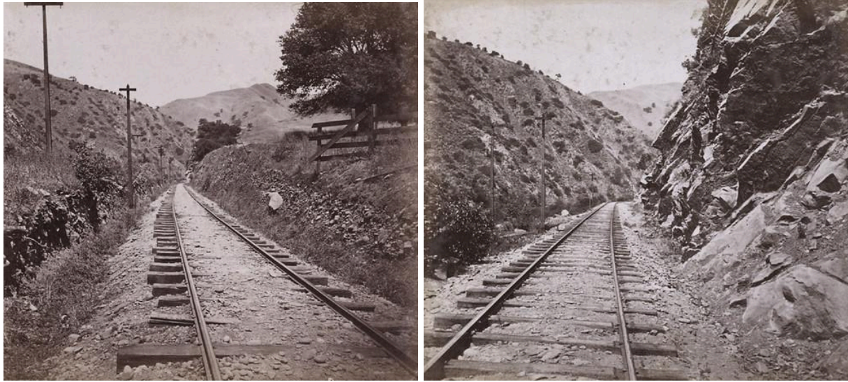
Fig. 11. (a) Left. Card 1524: Alameda Cañon, above Second crossing. (b) Right. Card 1525: Alameda Cañon, below Third bridge. Shows the original ruggedness of the through-cuts (left) and the rock-cuts (right) hand-carved by Chinese builders, pictured before growth of obscuring vegetation and widening of the cuts likely by machinery in the early 20th century. Images courtesy of the Society of California Pioneers, SCP-1253, SCP-1254.
